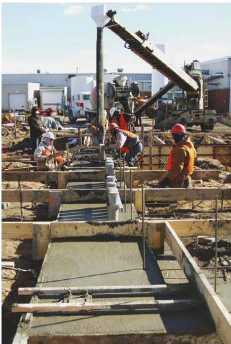
CASE IH turned to Lacy Construction once again.
