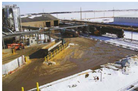
Pictured above: Nebraska Energy wet pit. At left: Truck scale and scale house.
